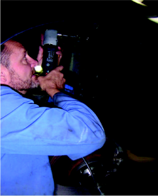
The author drilling the new upper fixing point
